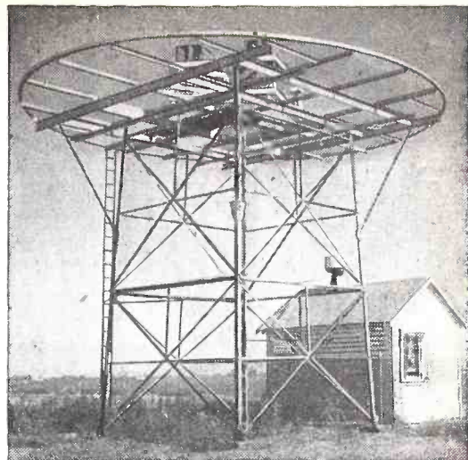
The 22-foot tower station and transmitter house for a very-high-frequency radio range.
